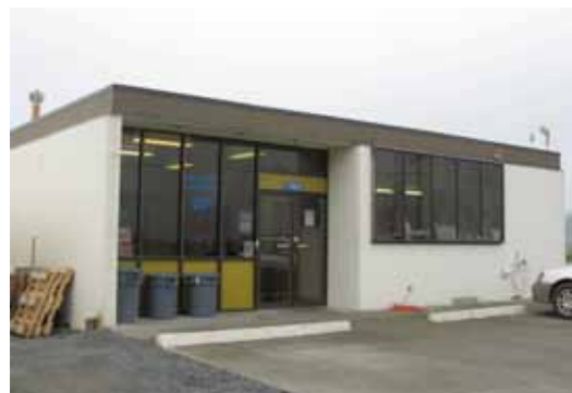
The IGFC Processing Center
