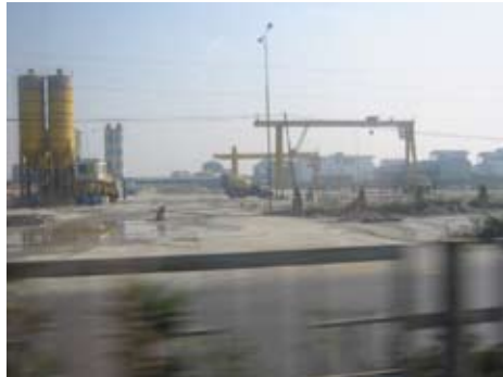
Bulk material handling, Red River Delta
