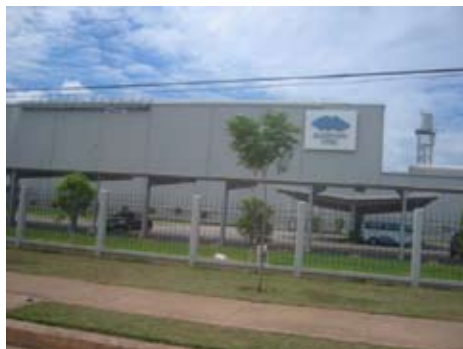
Bluescope Steel, Phu My plant
