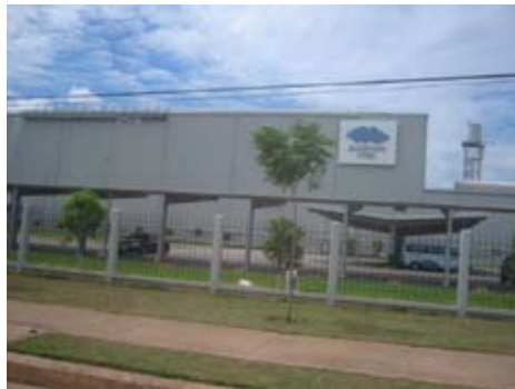
Bluescope Steel, Phu My plant
