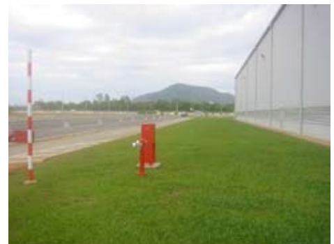
This area beside the Bluescope Steel Phu My Plant is notable because the adjacent road was built over a former minefield, which had to be de-mined and declared safe, before the road could be built. This is a problem often associated with building in former war zones. The de-mining and all road work was carried out and paid for by Bluescope Steel
