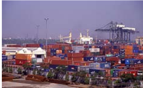
Cai Lan international container terminal
