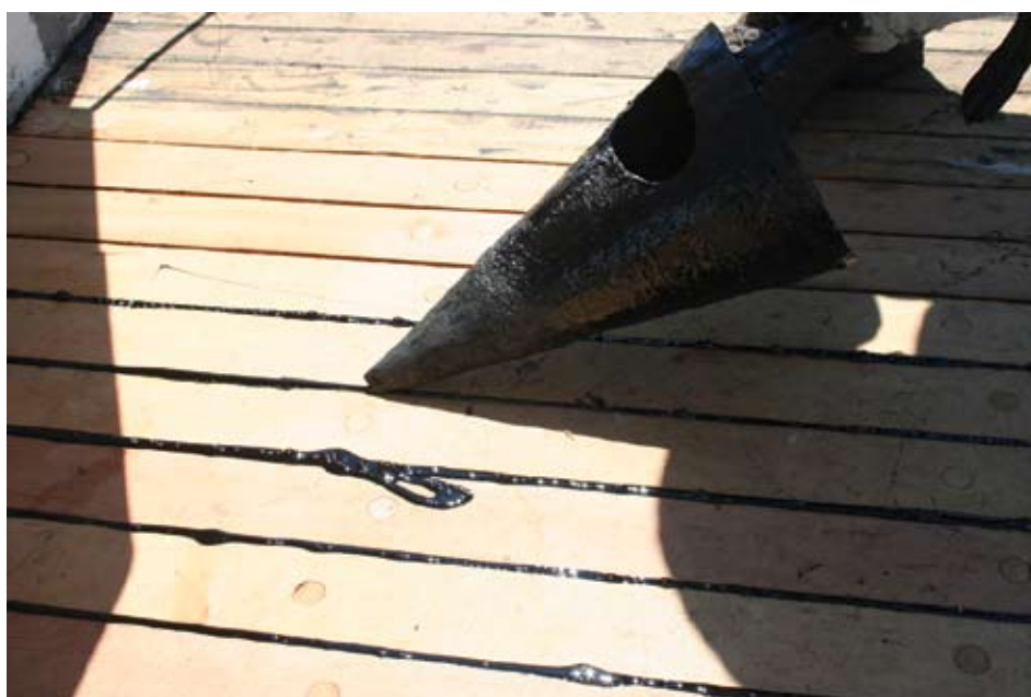
Pitch cone used to apply pitch to seam
