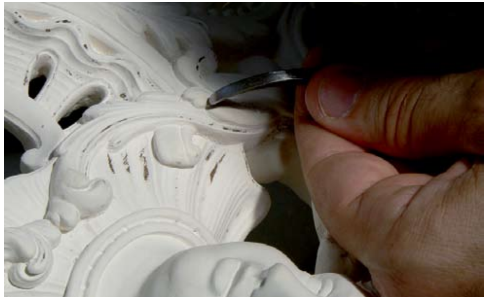
Figure 5: Repairer re-cutting gesso
