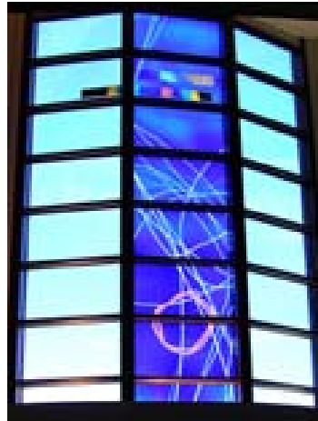
Excellent example of precision cutting & laminating of flashed glass with etched details. The work is installed in double glazed units
