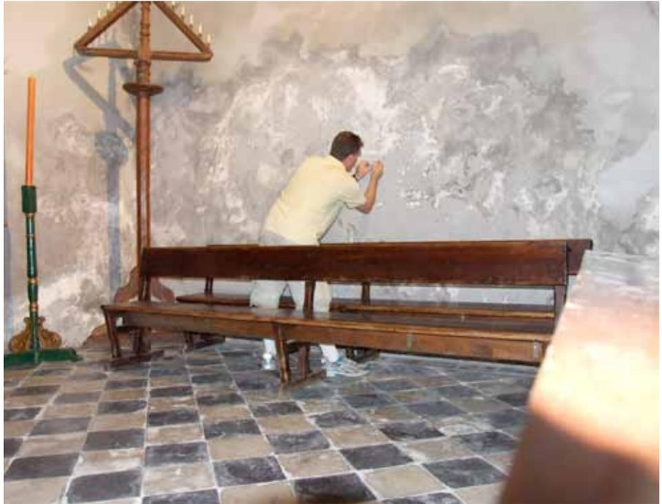
Figure 16. An example of penetrating damp
