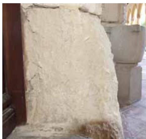
The field trial focused on the two major masonry units at the base of the jambs of the doorway to the chapel. The bases of both stones are in direct contact with the tiled surface of the cloister. The cloister would have been mopped daily by the monks and more recently by the nuns. A damp proof course of any description has not been incorporated into the structure (or may have been and has been bridged by subsequent increases of corridor levels).
