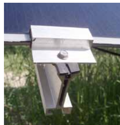
Clip & aluminium extrusion securing panel
