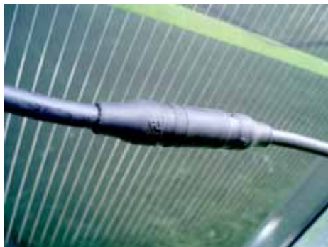
Snap-in weather proof PV panel connector
