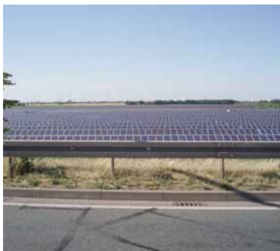
Solar array with CSG panels at rear
