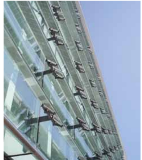
Solar panels used to shade shop windows
