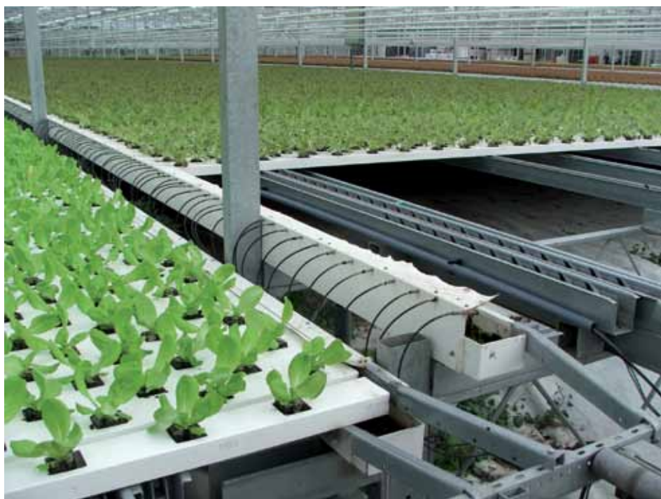
Moving gully system showing drip feed lines and drive system under gullies, Barendrecht, Netherlands
