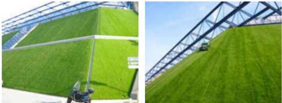
Ford Motor Plant – Dearborn, Michigan. The biggest green roof in the world at 10.4 acres
