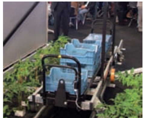
Transport Trolley used on heating pipes
