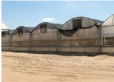
Greenhouse structures for trials
