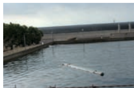
Water storage for heating system
