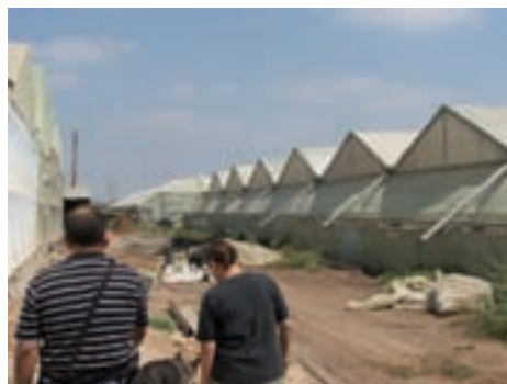
Straschnow Farm Greenhouse structures
