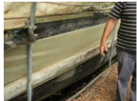
Pad and fan cooling system
