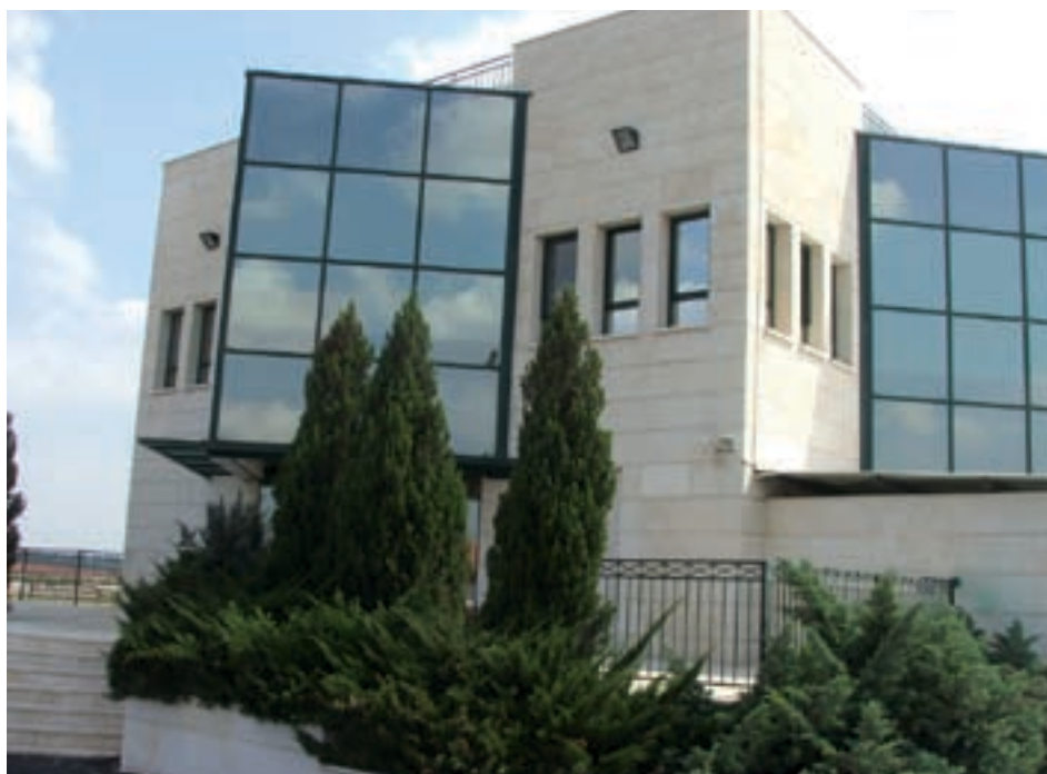
Hefer Association Water Management Facility
