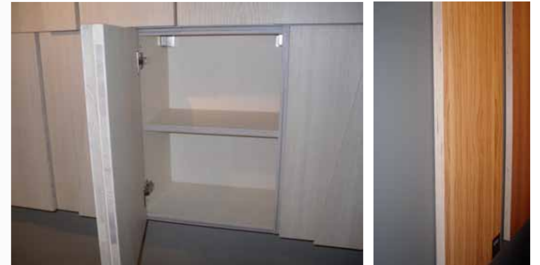
Core stock door with ply carcass
