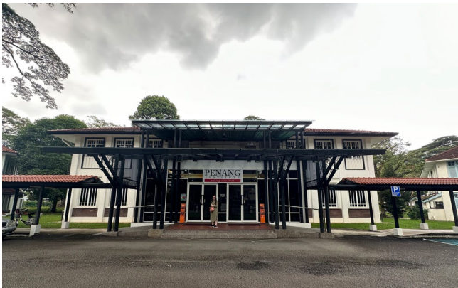
Figure 31. Penang Institute building
