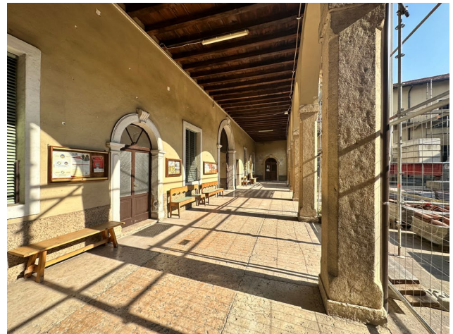
Figure 29. Outside monastery with construction
