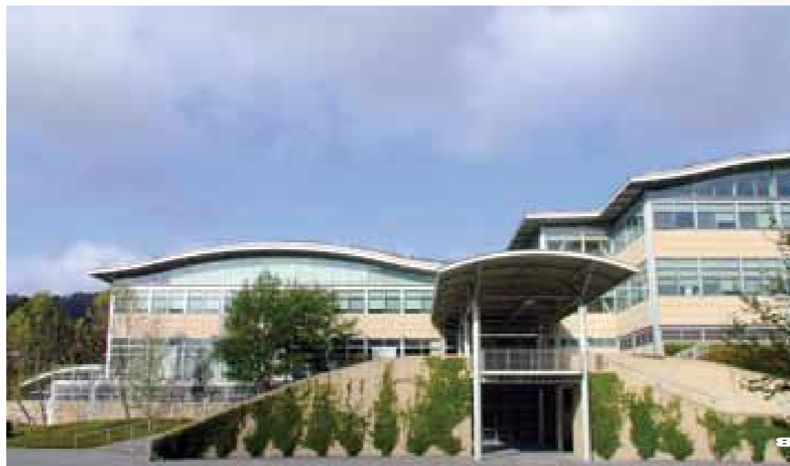
Front entrance of building
