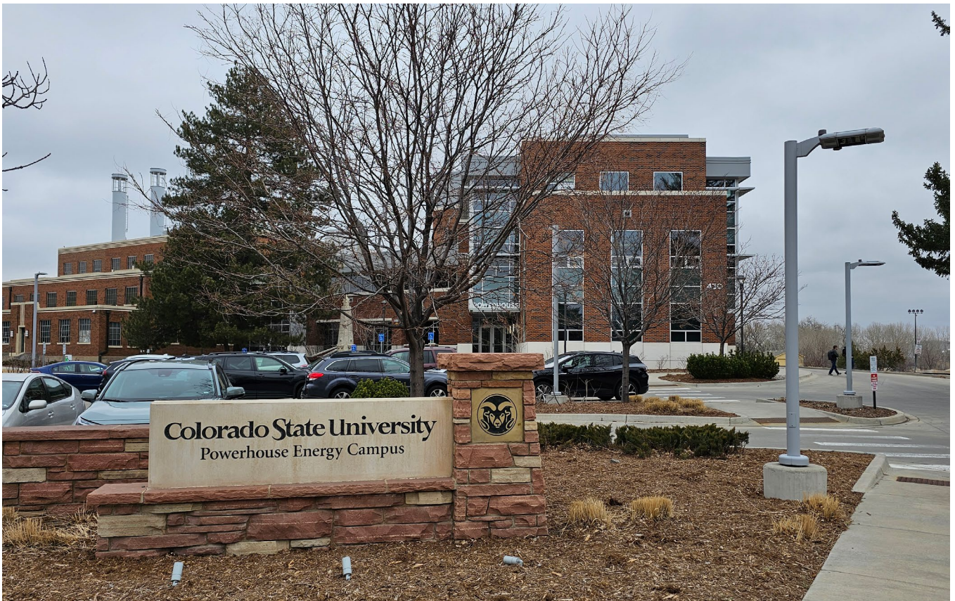
Figure 10: Image of the CSU Powerhouse Campus in Fort Collins. The vertical white columns protruding from the brick building are vertical wind turbines. An example of CSUs investigation into various renewable energy sources.
