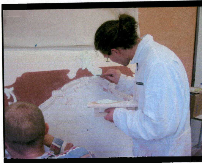
Application and carving of plaster. Venice Centre
