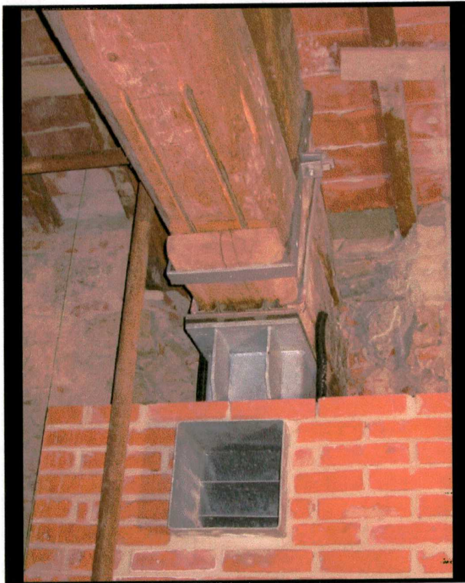
Steel Intervention. Villa Demidoff. Florence
