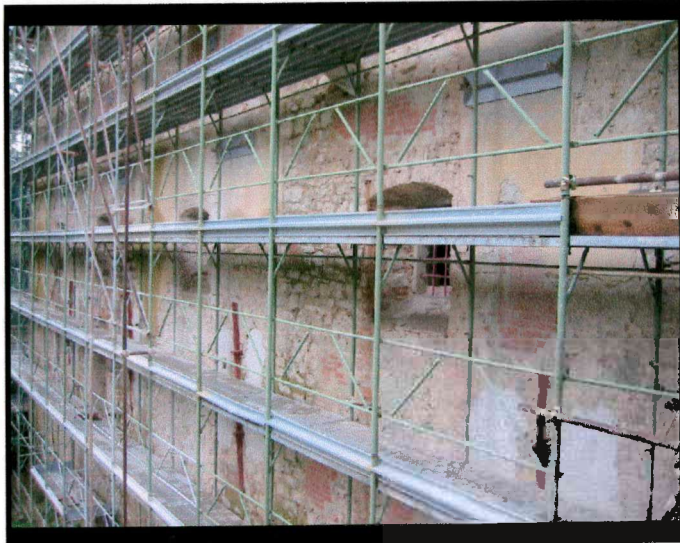
Façade restoration. Villa Demidoff. Florence.
