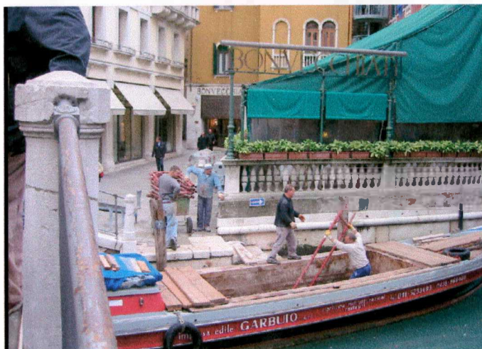
Scaffold delivery. Venice
