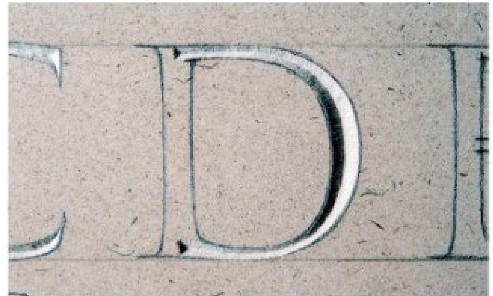
Detail showing V-incised alphabet in Portland limestone (Tom Perkins)
