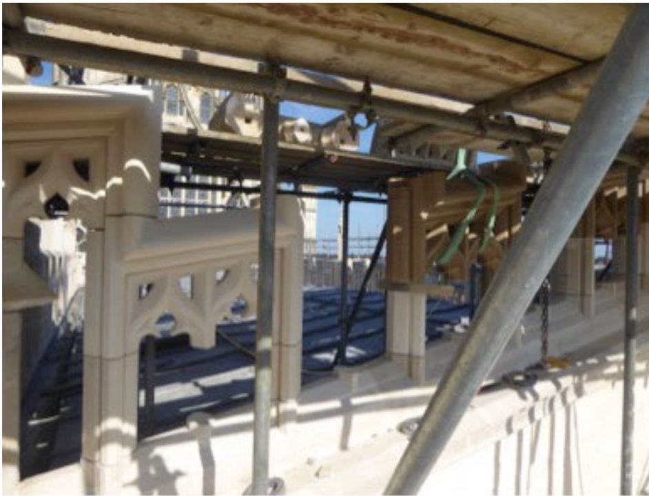
Partially installed open tracery merlots, Lady Chapel Parapet Balustrade (TH)
