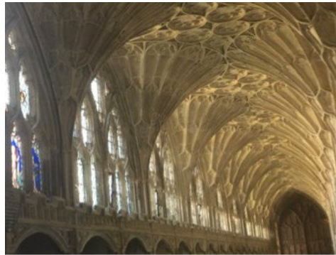
The exquisitely executed fan vaulting the cloister walk, arguably a high point in English masonry (TH)
