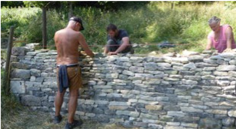
In unseasonably hot conditions workshop participants rebuilding both faces of the wall
