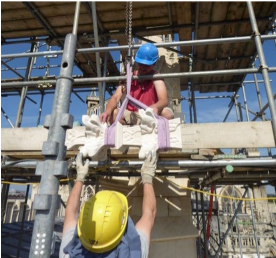
Raising the last stone to be fixed on the Lady Chapel Pinnacles (TH)
