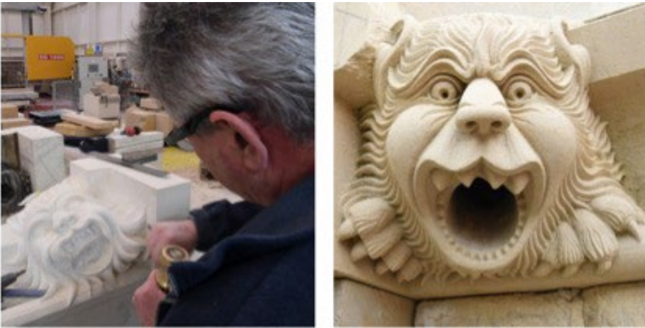
Left: Master carver prepares new guttering overflow gargoyle. Right: Recently installed piece (Canterbury Cathedral Trust)
