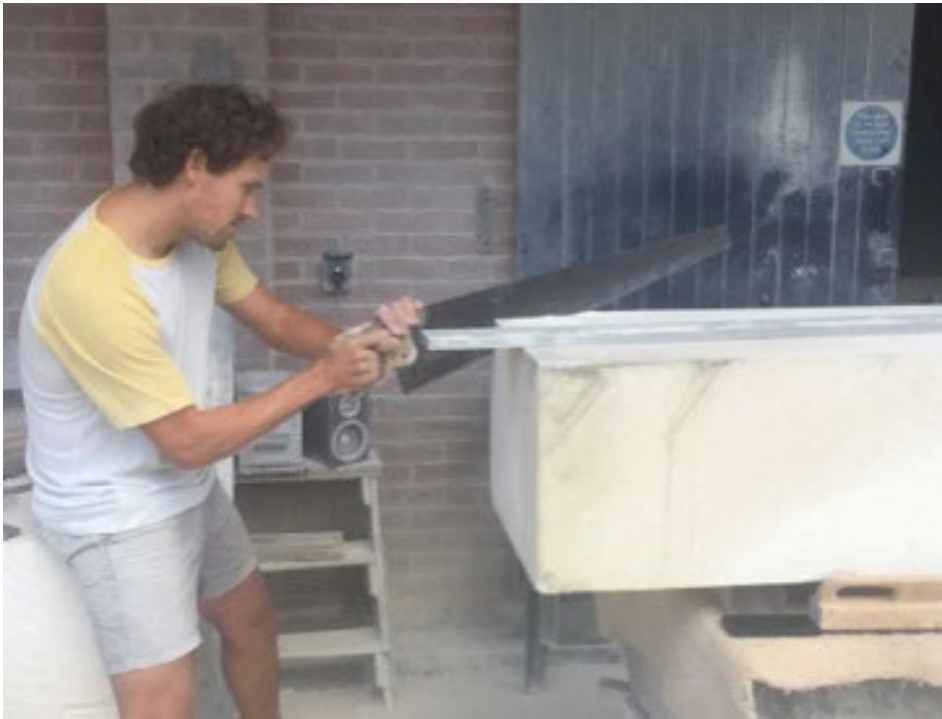
James commencing work on the merlot: the soft nature of the freshly quarried stone permitted James to cut a chamfer with a hand saw with 10mm wide teeth. (photo TH)
