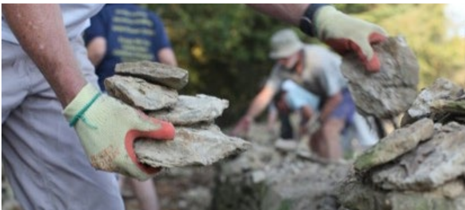
Careful selection of infill material to prevent rocking.(TH)
