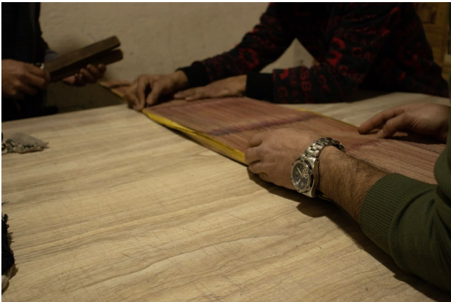
Figure 64. Decorative sunray held in place while it is fixed with wooden planks
