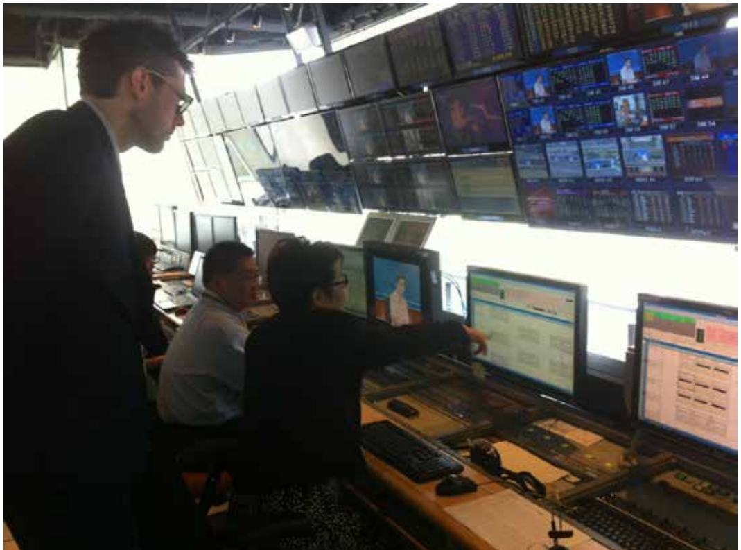
Control Room 2 Director area
