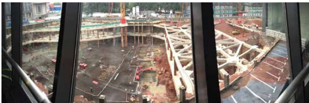
Nanjing Construction of new tower
