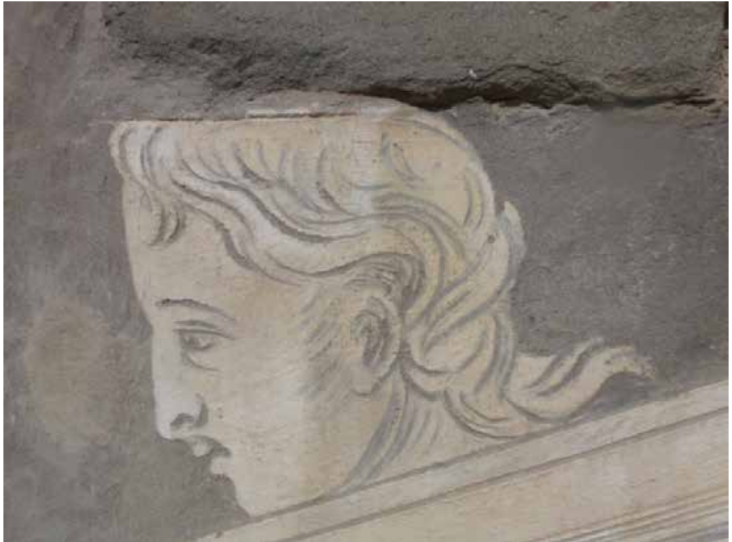
Detail of sgraffito work on the exterior of a building in Piazza dei Cavalieri, Pisa
