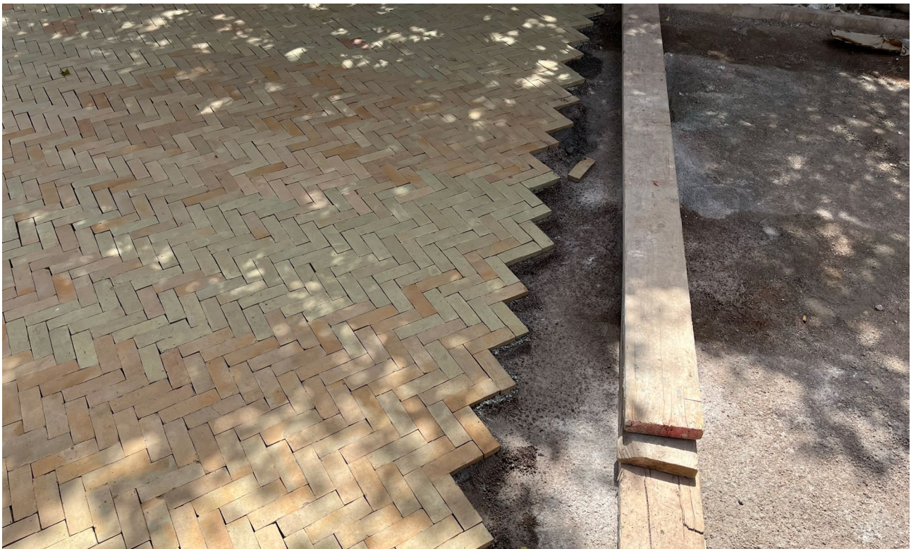
Figure 19. Streetscape construction - Marrakesh.
