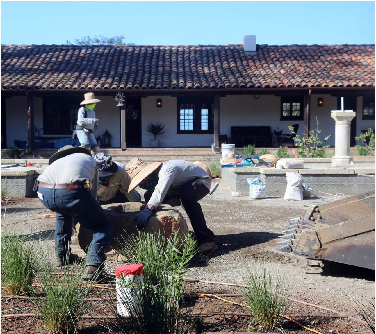
Figure 17. Private residence construction, Terremoto - Los Angeles, CA.
