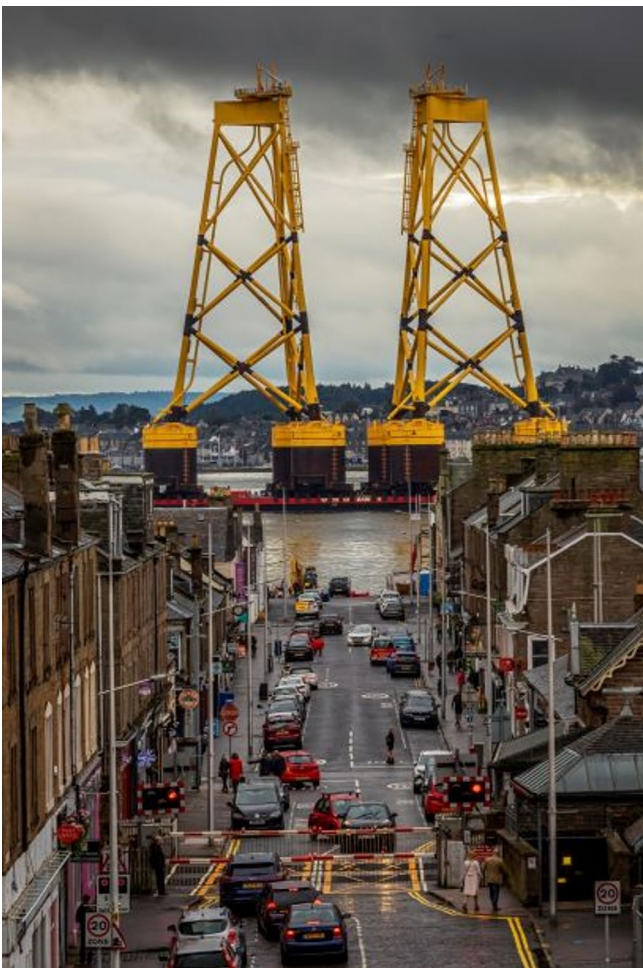
Figure 10. Foundation Jackets leaving the Port of Nigg on their way to the Seagreen Offshore Farm.
